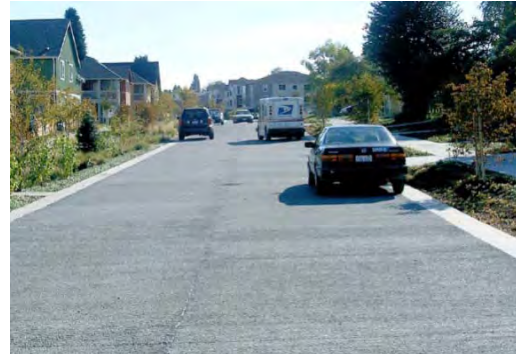
Figure 29: Seattle's First Pervious Pavement Street Source: www.usbg.gov/education/events/loader.cfm?csModule=security/getfile&pageid=29114
