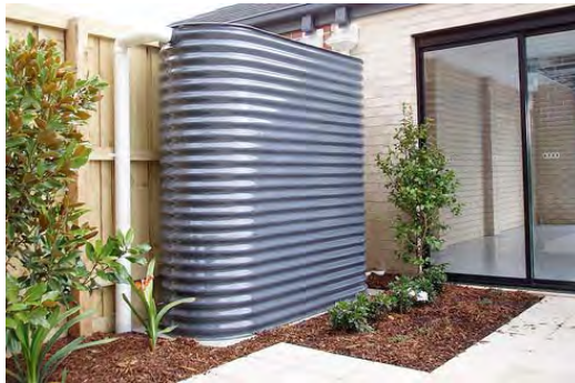
Figure 30: Rainwater Harvesting Tank
