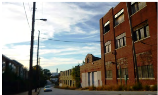
Figure 11: New residential project in the Pittsburgh neighborhood and fire-damaged industrial buildings
