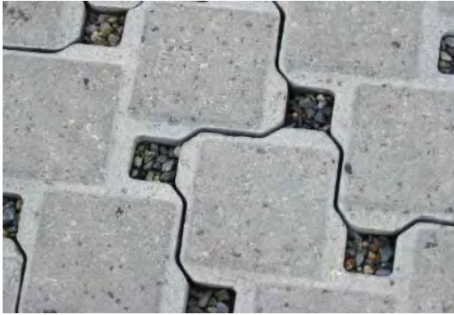
Figure 28: Pervious Walkway Source: www.usbg.gov/education/events/loader.cfm?csModule=security/getfile&pageid=29114
