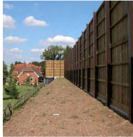
Figure 18: Acoustic buffer Source: http://betaacousticbarriers.co.uk
