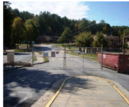
Figure 5: The recently decommissioned public homes provide new land to expand and intensify the industrial productivity of AIP
