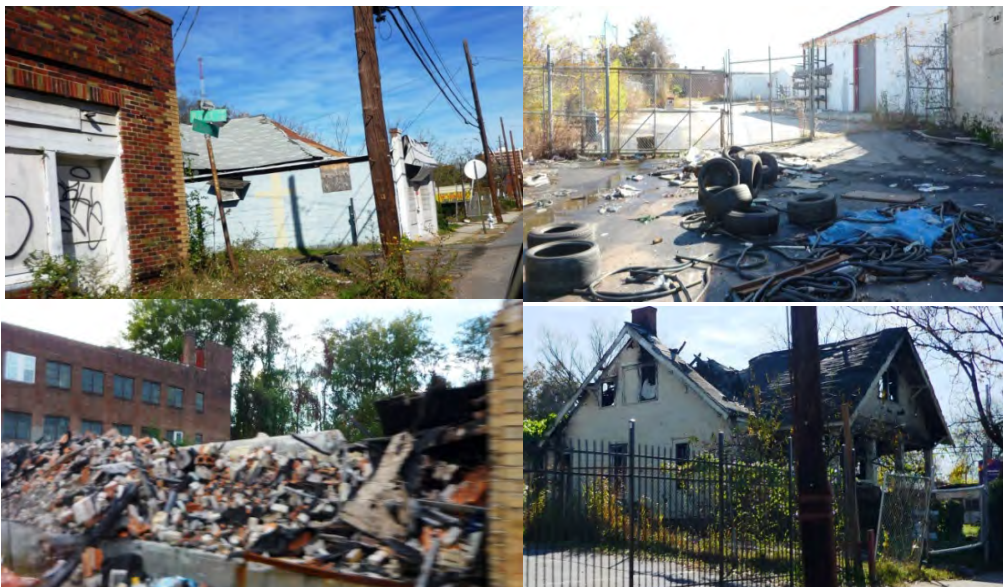
Figure 10: Dilapidated buildings, illegal dumping, demolition debris, and fire-damaged houses located in Metropolitan Corridor North Node
